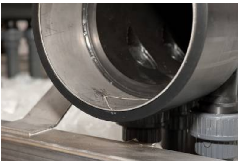
Figure 6.3.12.1b: Header Insert for Straub-Flex.
