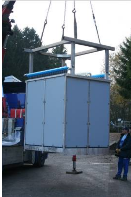
Figure 6.3.11.1: Module prior to installation in the membrane tank.
