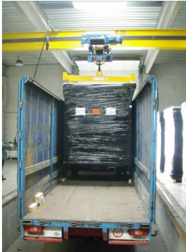
Figure 6.3.9.1a: Module removal with special lifting frame.
