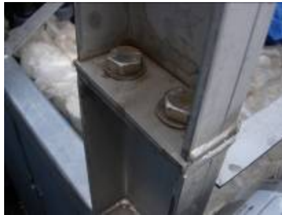
Figure 6.3.8.2: Leg connection to PSH 1800 module frame
